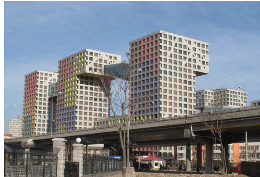
Contemporary MOMA in Beijing China - Steven Holl Architects
